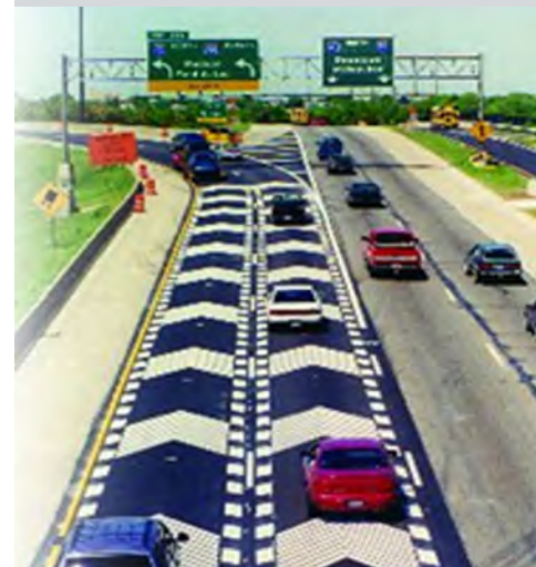
Photo showing chevron pattern painted on the roadway, to promote speed management amongst automobile drivers by Wisconsin DOT. Image source: https://www.forconstructionpros.com/pavement-maintenance/marking-striping/article/10117519/stripping-for-safety .
